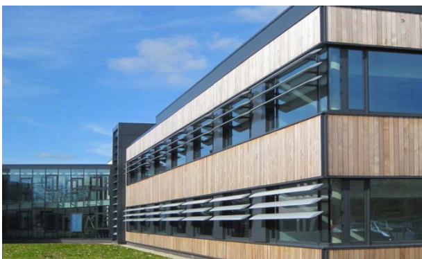
Centre for Ecology & Hydrology A new laboratory designed to achieve a BREEAM 'Excellent' environmental assessment.
